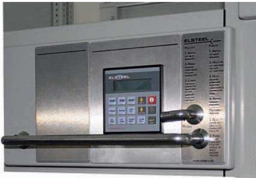
Elsteel MOTOR VISION is a simple low cost multi-function controller that provides motor starting and control functions with communications.
